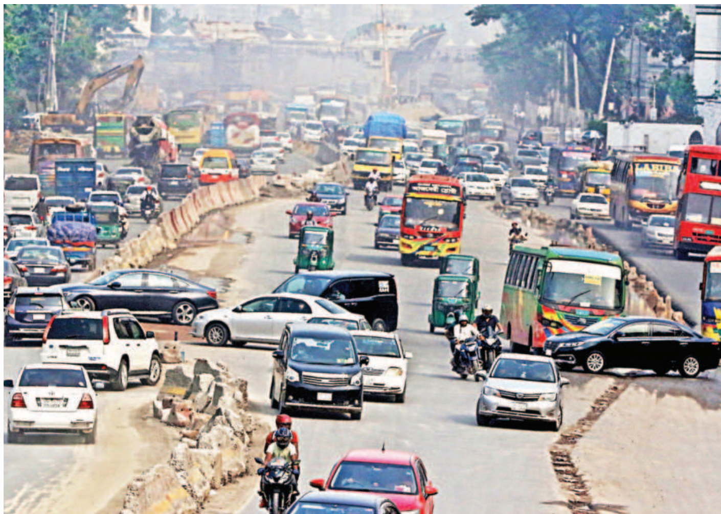
With the dividers being broken down, and no one to monitor traffic movement, vehicles were seen taking advantage of the situation, by taking U-turns towards Tongi and Airport Road. As this road at Uttara's Azampur area usually remains busy with large vehicles, this situation is creating gridlocks and poses risks for accidents. This photo was taken yesterday.
