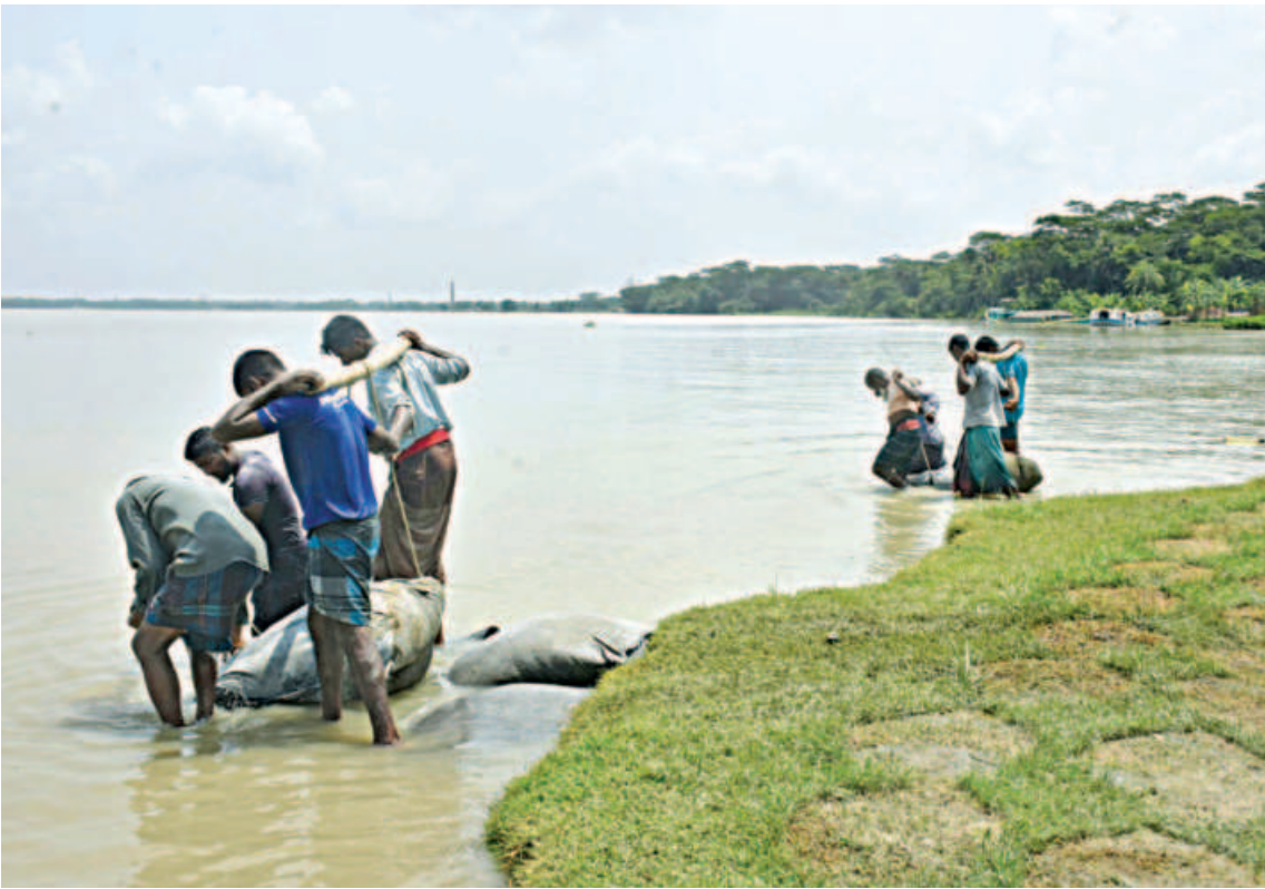
Labourers dump sandbags in the Sugandha to protect the bank from erosion in Jhalakathi's Nalchhiti upazila yesterday. The swelling river is threatening arable land and people's homes and business there.
