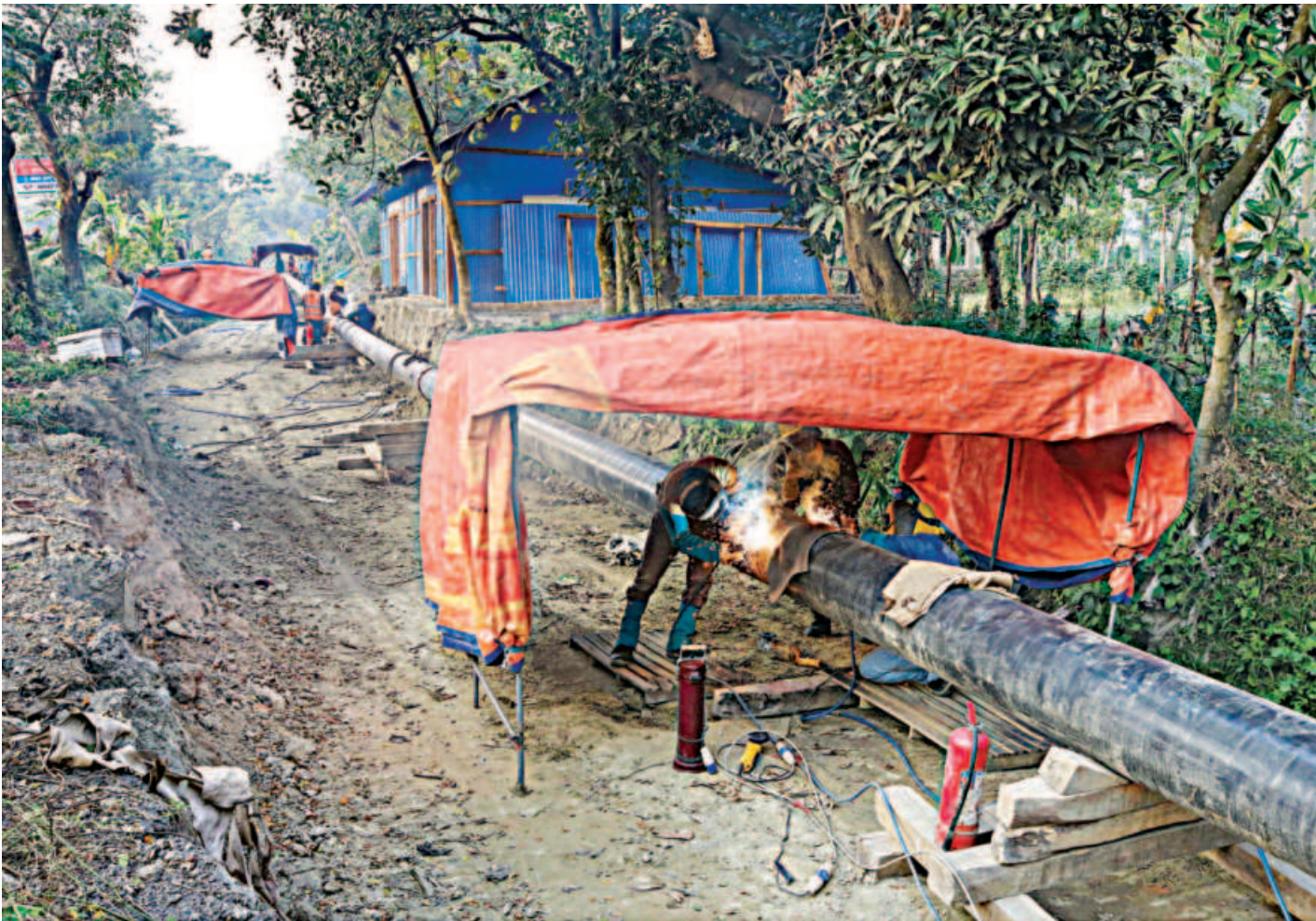
Workers are seen welding together two sections of the 250-kilometre fuel pipeline between Chattogram and Dhaka. Being implemented at a cost of about Tk 3,172 crore, the project is scheduled to be complete by this December. The photo was taken in Sitakunda upazila of Chattogram recently.
