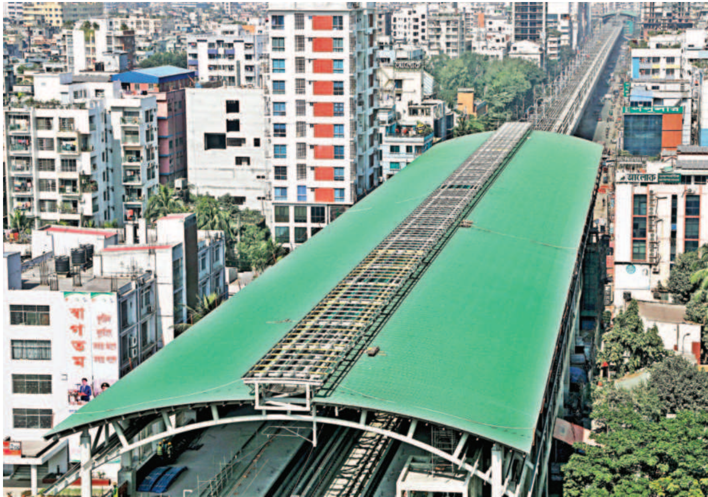
A partial view of the metro rail project in the capital. Economists have called for caution during the years of 2027 and 2028 when Bangladesh will start paying interest due on four or five foreign loans taken for some mega-projects.
