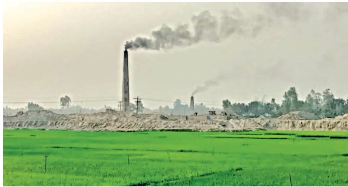
Thanks to the inaction of the concerned authorities, 130 illegal brick kilns have been operating in 14 upazilas of Lalmonirhat and Kurigram. In this photo, a brick kiln is seen emitting fume near a cropland in Mogholhat union of Lalmonirhat Sadar upazila.
