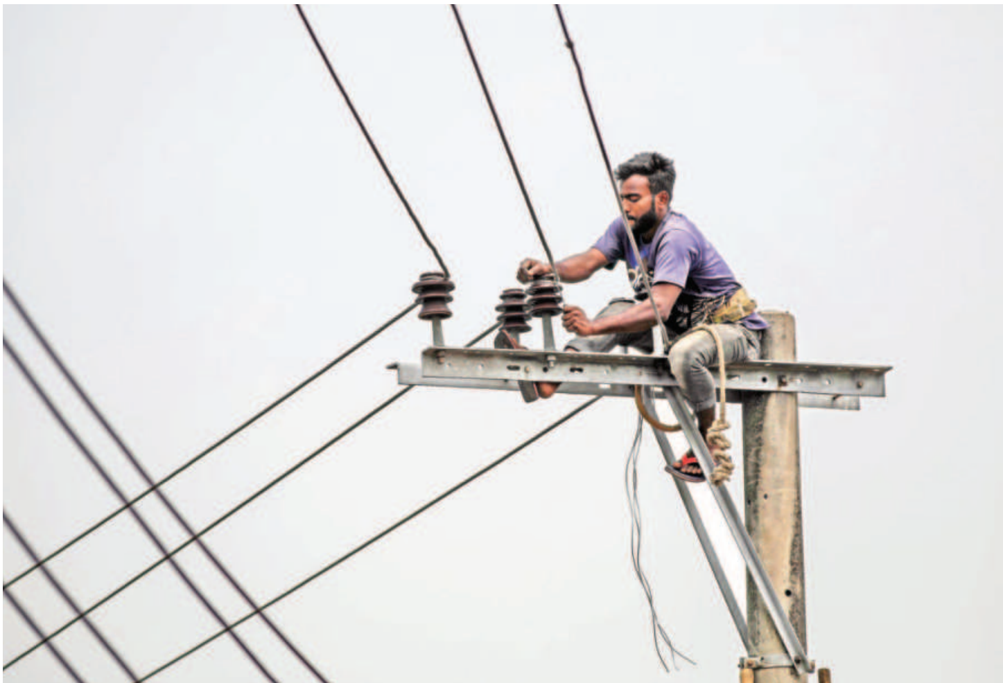
Sitting on a pole, a precariously positioned man repairs power lines in Chattogram city's Uttar Kattali area yesterday. He has a waist harness but it seems it is not tethered to anything. He also does not have any helmet.
