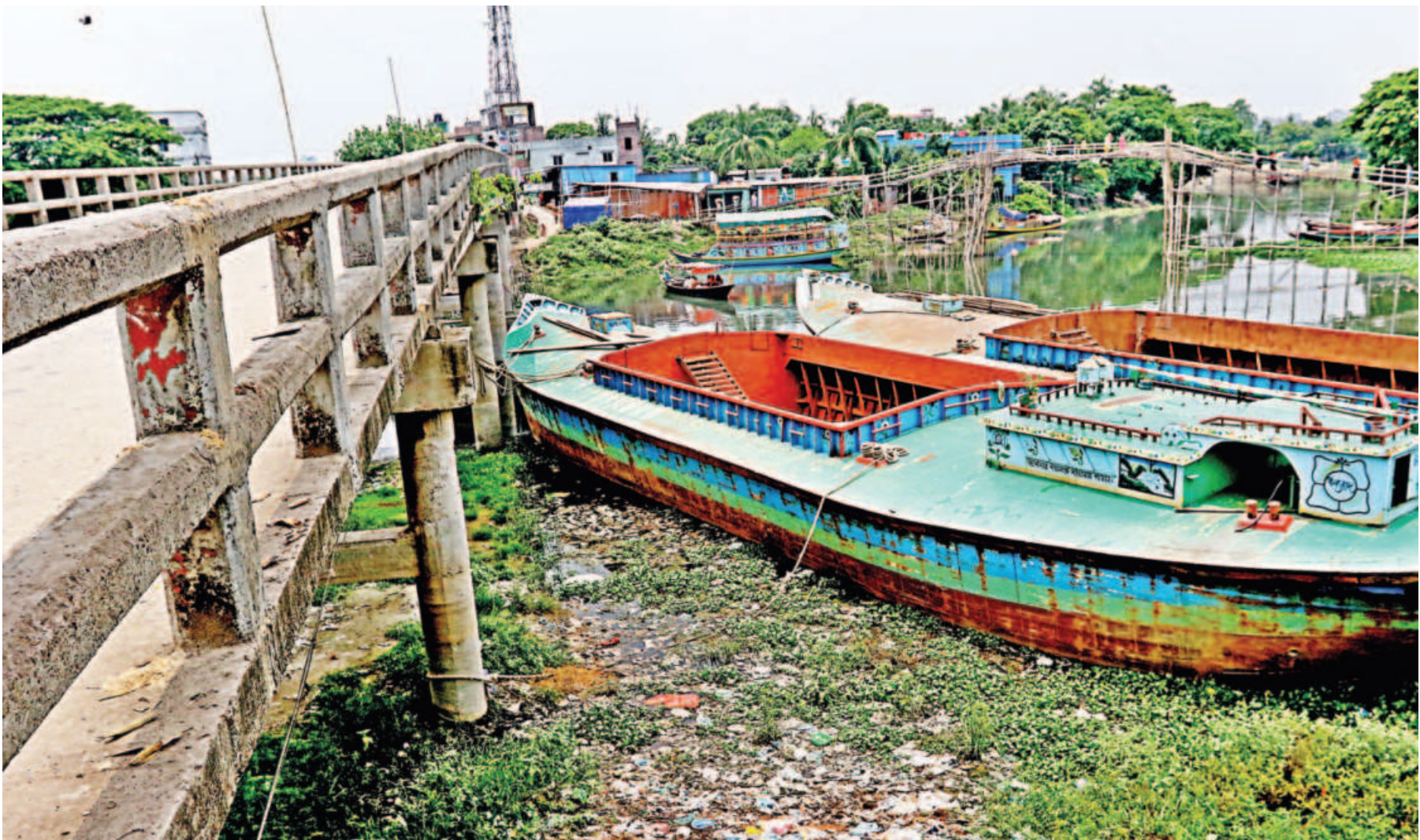
Large vessels are tied to the pillars of a bridge at Trimohony, Khilgaon, in the capital. Civil engineers say this practice can damage the bridge because the pillars are not designed to withstand the pull of such vessels.
