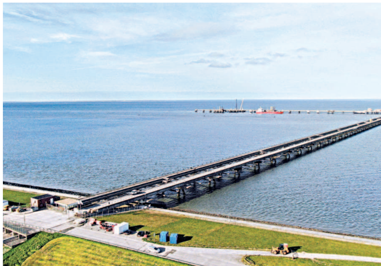
An aerial view of a pier for a planned floating liquefied natural gas (LNG) terminal in the harbour in Wilhelmshaven, Germany on May 4.
