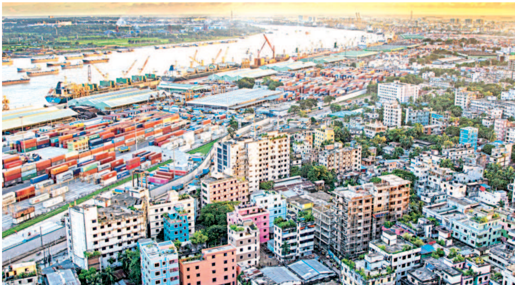
Work is ongoing to enhance the capacity of the country's premier sea port to handle more cargo and containers, officials said.
