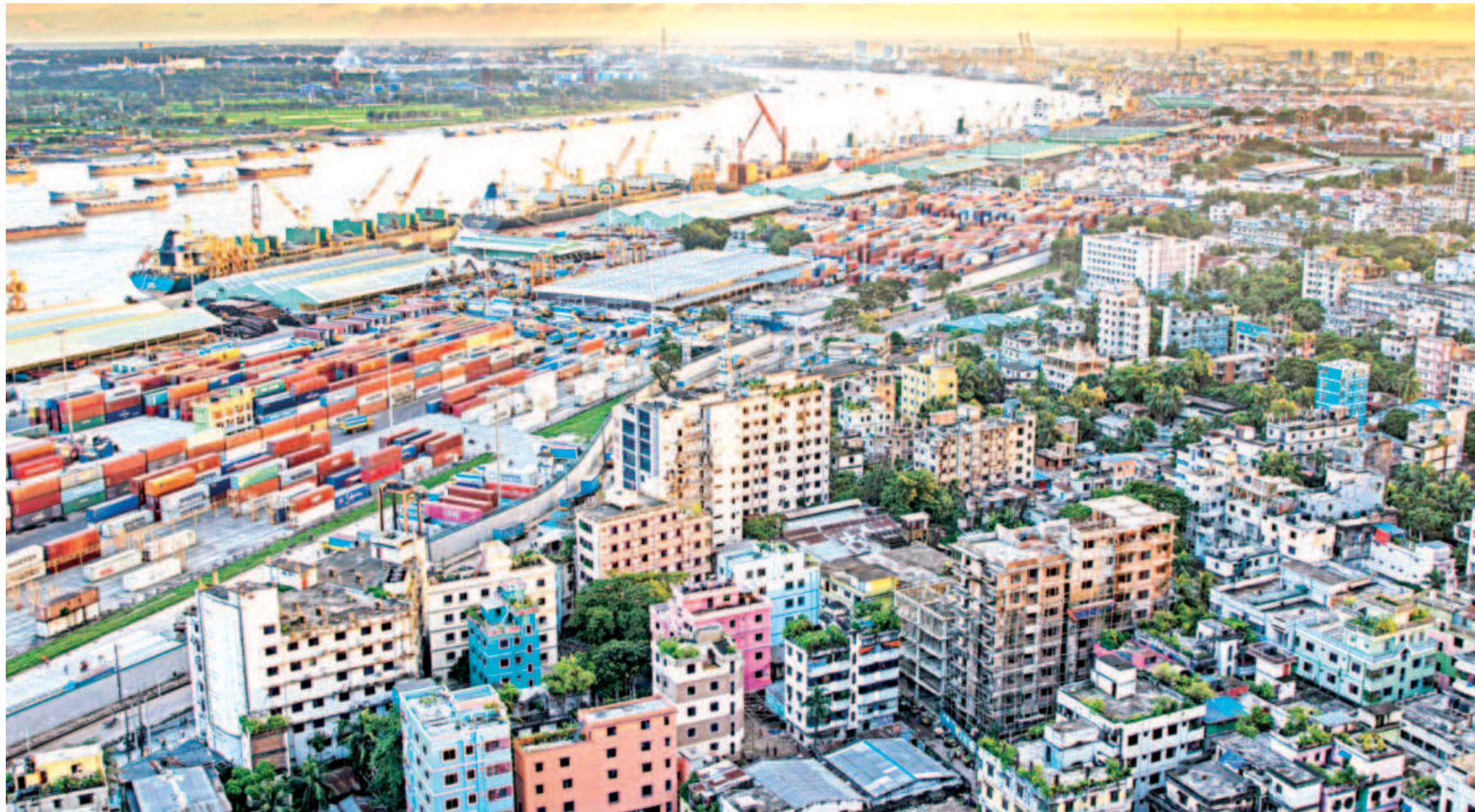
Work is ongoing to enhance the capacity of the country's premier sea port to handle more cargo and containers, officials said.
