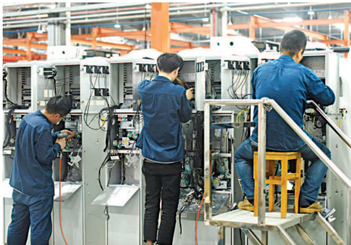
Workers assemble power distribution cabinets at a site in Hangzhou in eastern China's Zhejiang province. The International Monetary Fund has cut its growth forecast for China this year to 4.4 per cent, well below Beijing's target of around 5.5 per cent.
