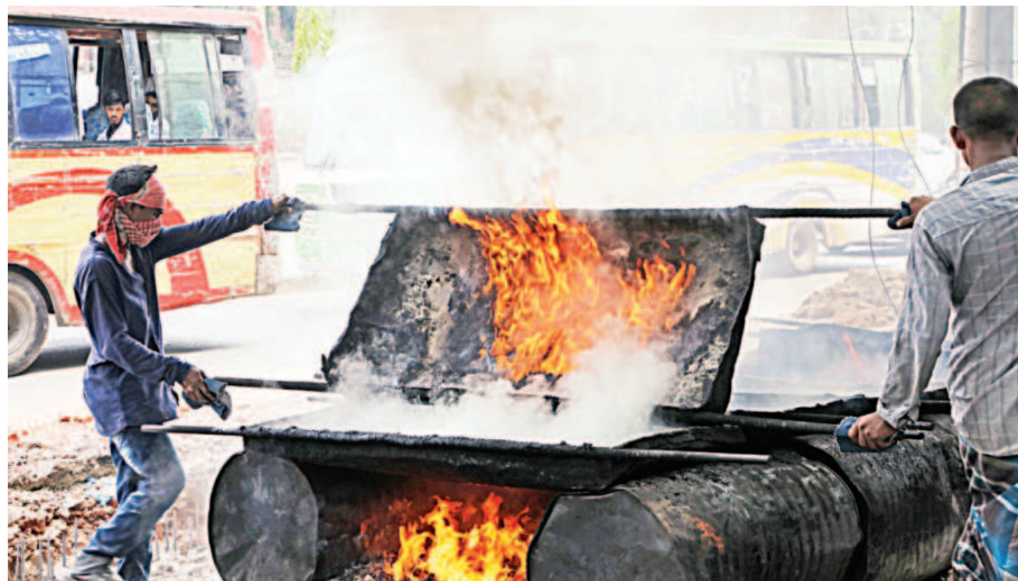
With no safety gear on and no masks to protect them from the fumes, workers are busy melting asphalt for the city's road construction work in an extremely hazardous environment. This photo was taken at the capital's Agargaon yesterday. PHOTO: PALASH KHAN
