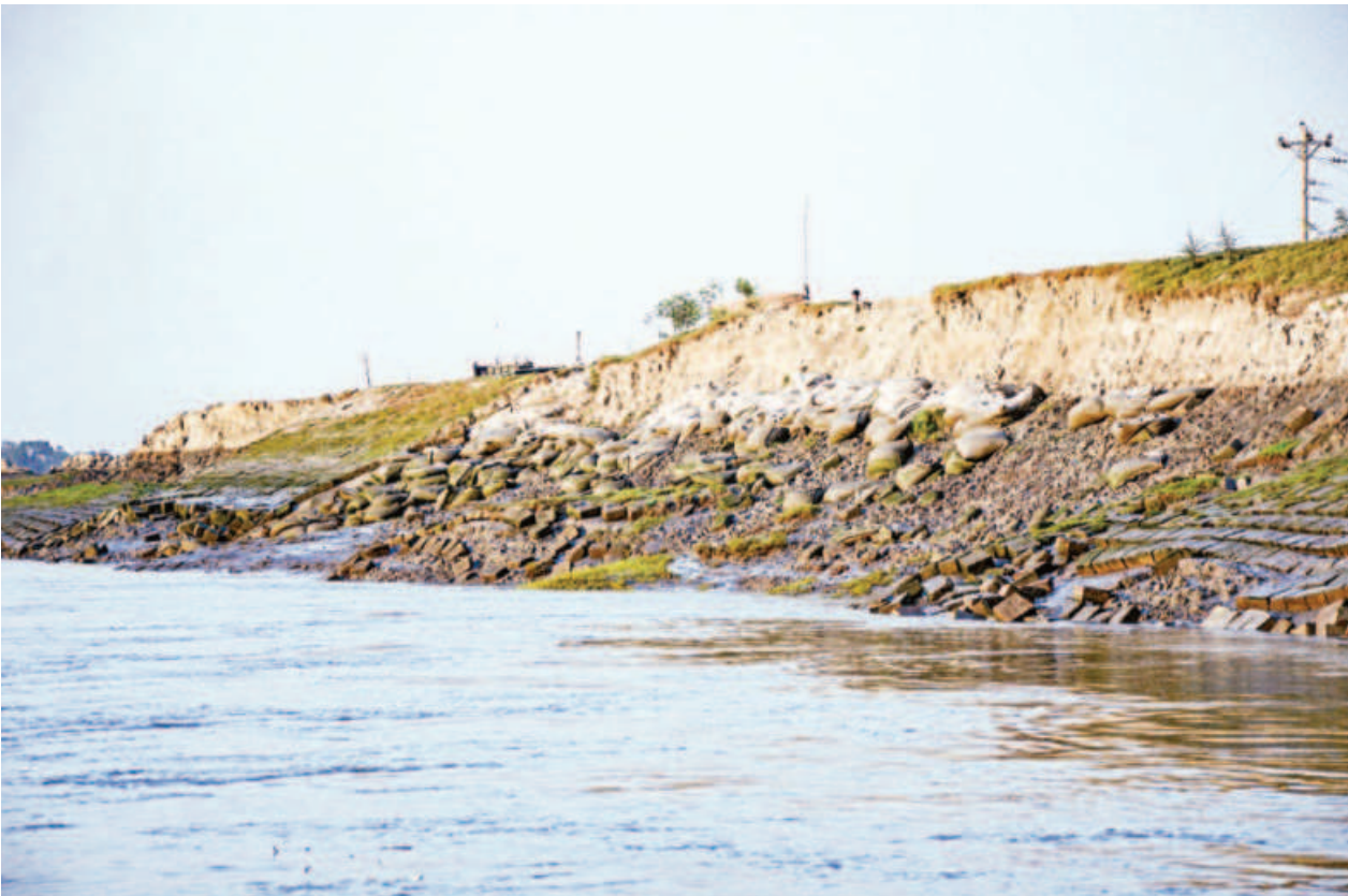
Blocks and geo bags dumped to protect an embankment in Noliyan area of Khulna’s Dacope upazila are in dilapidated condition. In the aftermath of Cyclone Aila in 2009, the authorities went for the block dumping, but years of neglect has turned them this way, posing risk of erosion.
