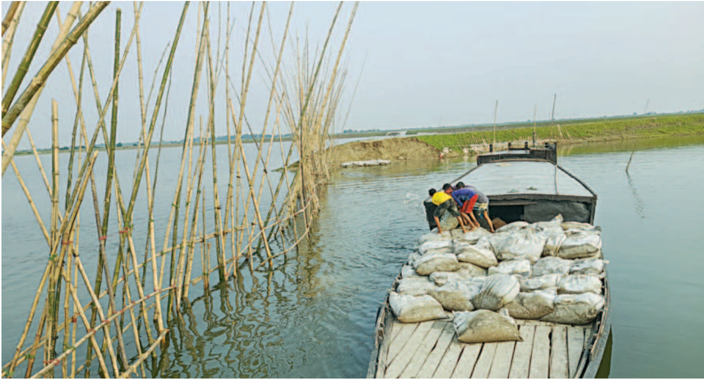
The staffers of Water Development Board dropping sandbags in the Kangsha river to fix the Dubail dyke in Sunamganj’s Dharmapasha upazila that gave way to flooding. The photo was taken yesterday.
