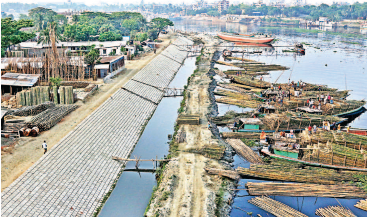
The Bangladesh Inland Water Transport Authority is building paved embankments along both banks of the Shitalakkhya river to make walkways and prevent erosion and encroachment in the Kanchpur area of the capital. The place is also popular among traders who bring bamboos from different parts of the country using the waterways.
