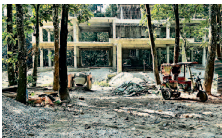
The construction of a two-storey rest house is underway on another land adjacent to where the artificial lake is supposed to be dug.
