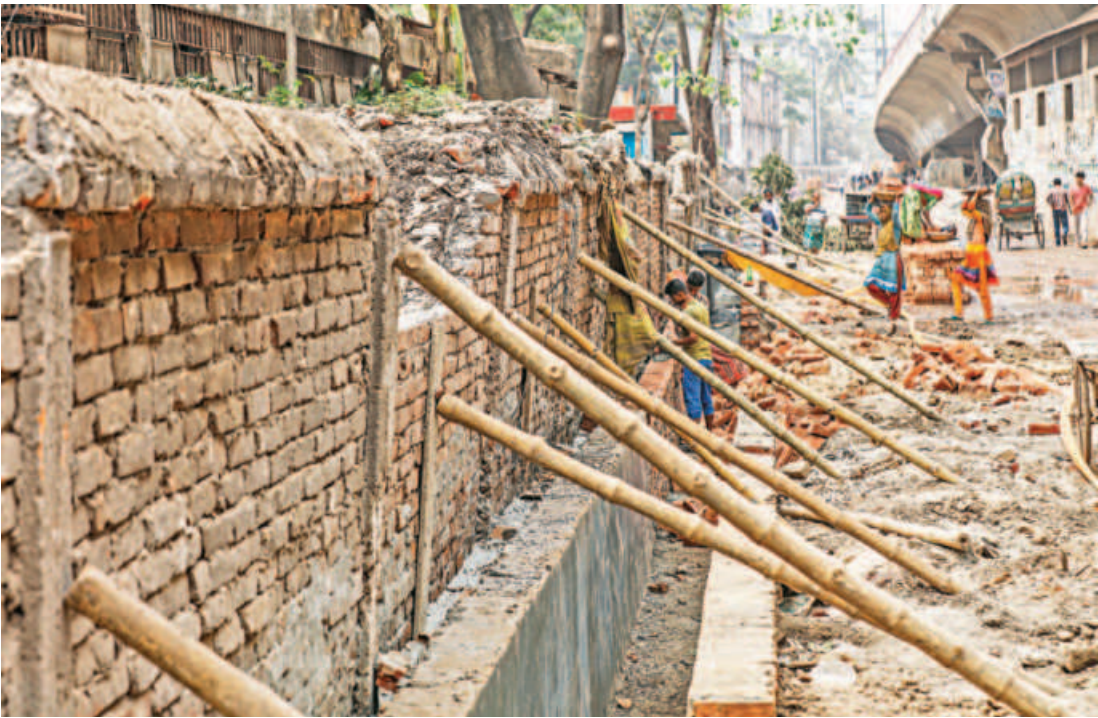
Construction works for a drain are ongoing right outside the boundaries of Central Veterinary Hospital on Old Dhaka’s Kazi Alauddin Road. However, as the walls of the hospital have become weaker due to the works, DSCC decided to precariously balance them on a few bamboos.
