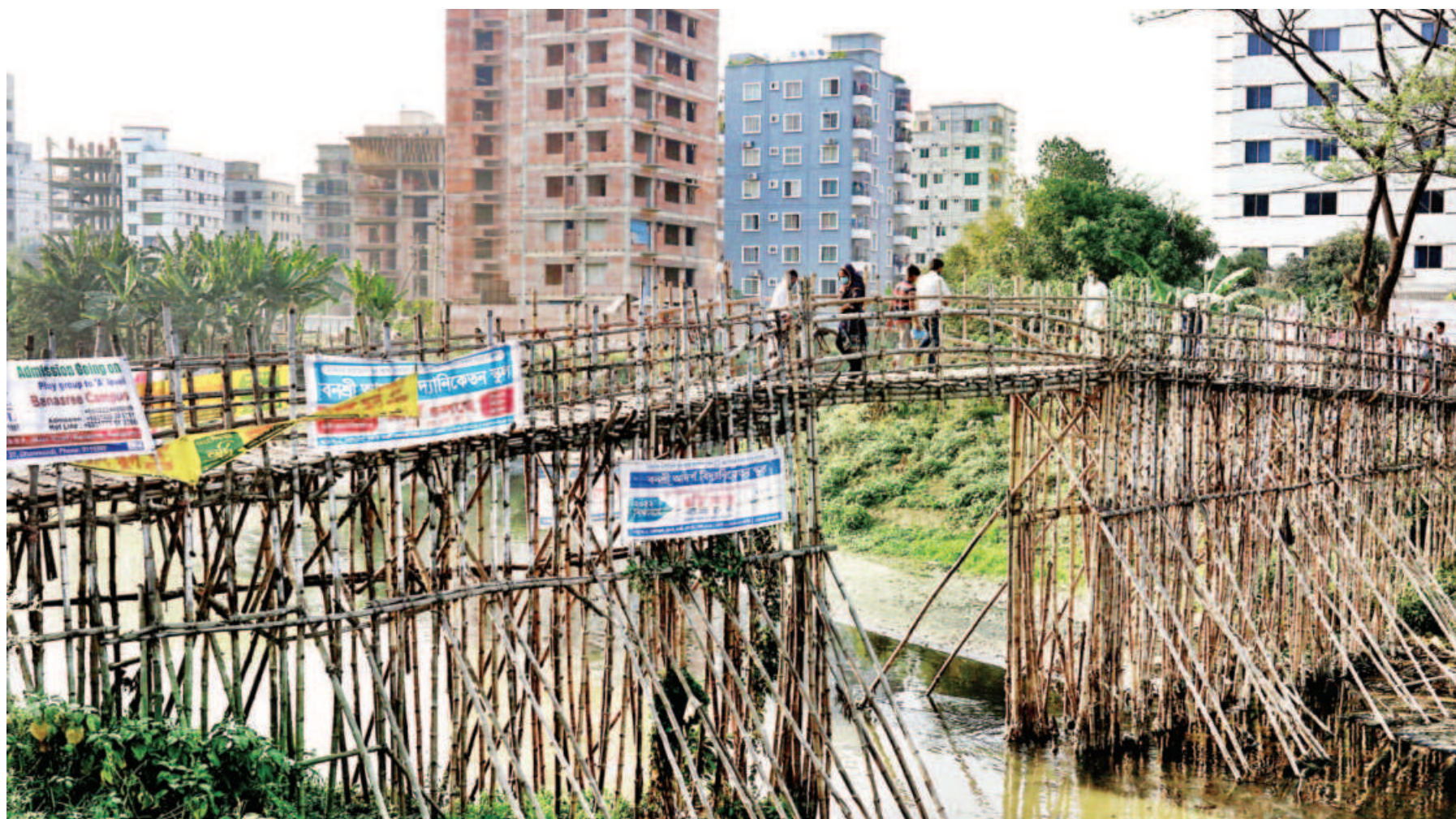
In the absence of this bamboo bridge that connects Banasree and Aftabnagar, one would have to make a journey of at least a kilometre and a half around Rampura. Sensing this, residents of housing societies from both sides agreed to build this bridge to save commuters from all that trouble. What's even more interesting is that the bridge falls right on the border of the two city corporations, as Banasree falls under DSCC and Aftabnagar under DNCC.
