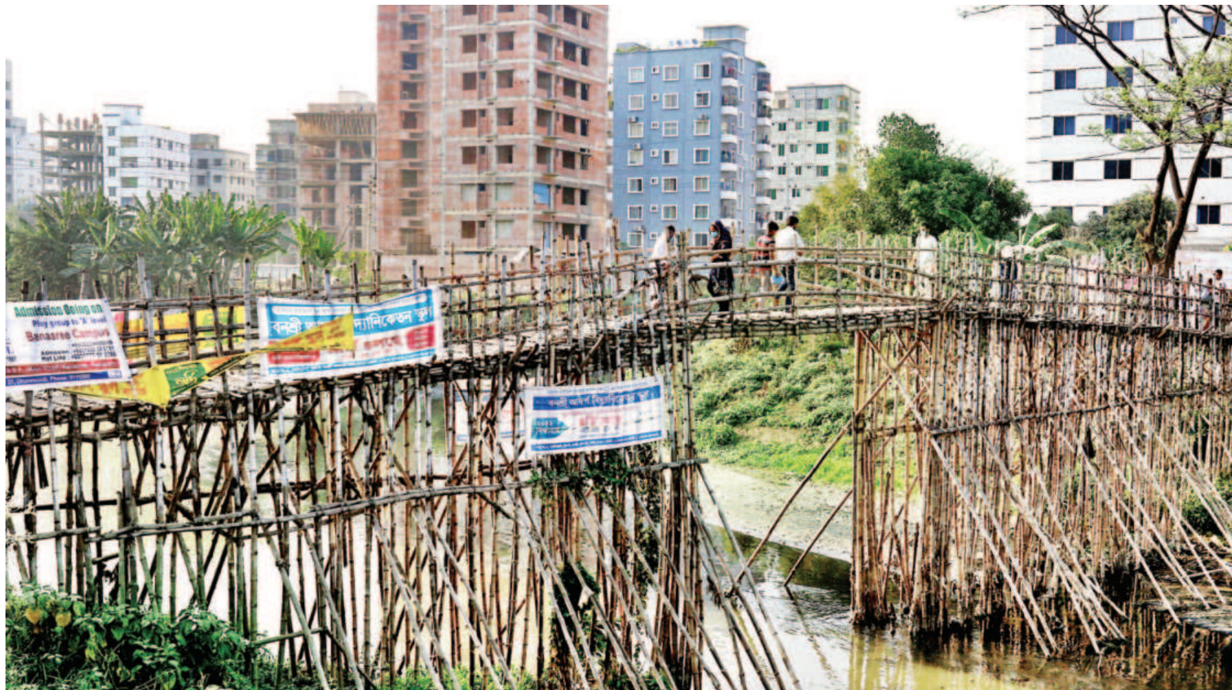
In the absence of this bamboo bridge that connects Banasree and Aftabnagar, one would have to make a journey of at least a kilometre and a half around Rampura. Sensing this, residents of housing societies from both sides agreed to build this bridge to save commuters from all that trouble. What's even more interesting is that the bridge falls right on the border of the two city corporations, as Banasree falls under DSCC and Aftabnagar under DNCC.
