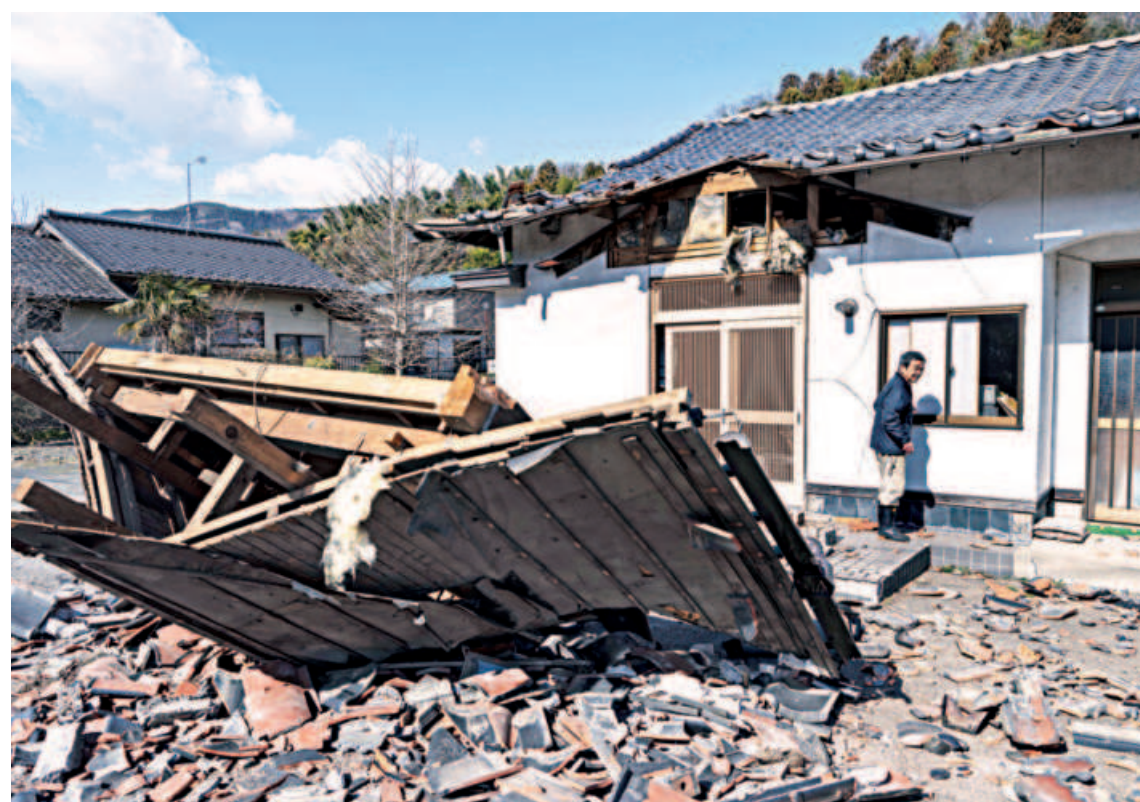
A man walks in front of his damaged restaurant in Shiroishi, Miyagi prefecture yesterday, after a 7.3-magnitude earthquake jolted east Japan the night before. The tremor left thousands of homes without water and power. At least two people died and 161 were injured.
