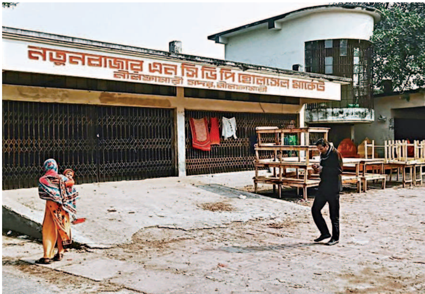
The Notun Bazar NCDP Wholesale Market in the sadar upazila of Nilphamari has been shuttered for years as farmers and wholesalers did not use it for their lack of knowledge about modern marketing systems. The market was set up to help growers receive fair prices for their produce. The photo was taken recently.
