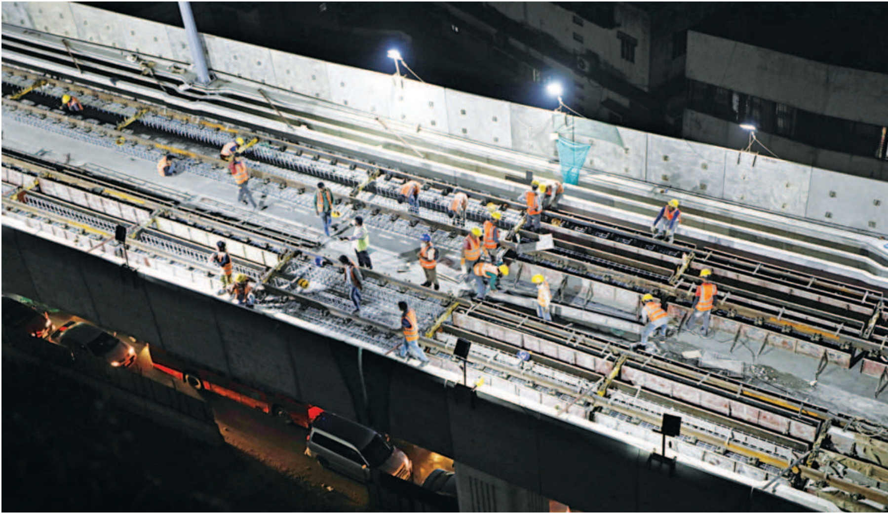
Illuminated by bright spotlights, workers in high visibility vests and hard hats stand in stark contrast to the surrounding darkness as they install tracks on the viaduct of the metro rail project at the capital’s Kazi Nazrul Islam Avenue. The photo was taken around 7:30pm yesterday, and they usually work deep into the night to ensure timely completion of the project.
