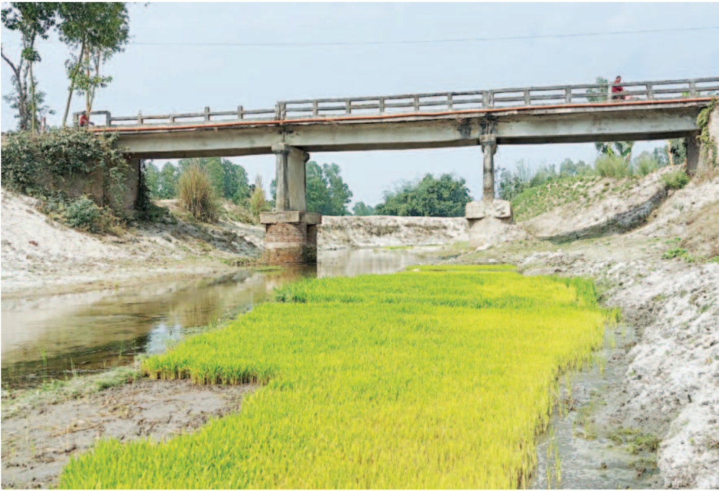
As the excavation works weren't done thoroughly enough, something that locals blame on the contractors of the project, this channel of the Suk river has filled up with silt and sand and been turned into a farmland for cultivating crops and vegetables.
