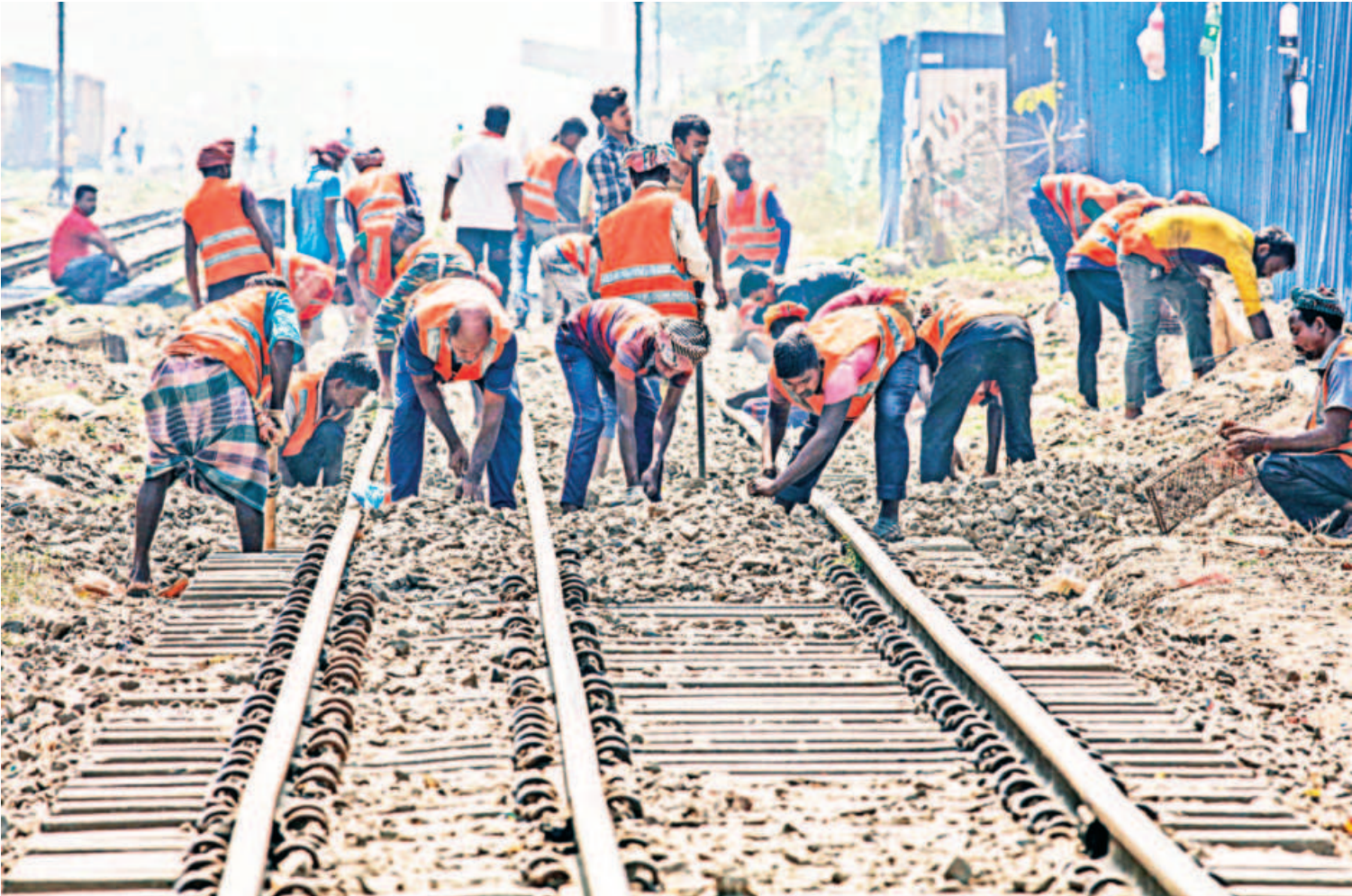
Debris, such as rocks and discarded materials, that have slipped within railway sleepers can lead to grave danger as speeding trains rush over them. To avert accidents of this kind, workers have been hard at work at the Tejgaon rail crossing, cleaning each section of the line with caution. This photo was taken yesterday.
