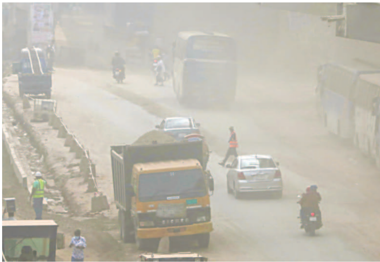
A blanket of dust covers the Tongi Bazar bus stop area in Gazipur as part of the Dhaka-Mymensingh highway is dug up for implementing a development project. The photo was taken recently.
