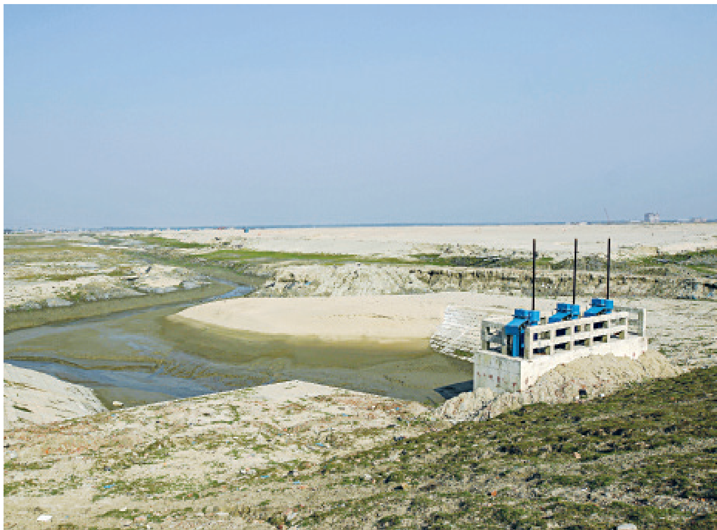
A view of the Daborkhali canal in Chattogram's Ichakhali union reveals that large portions of the water body have been filled up. Bangladesh Export Processing Zone Authority filled up a two-km stretch of the canal, the health of which is critical for irrigation as well as preventing waterlogging, to set up an economic zone. The photo was taken recently.
