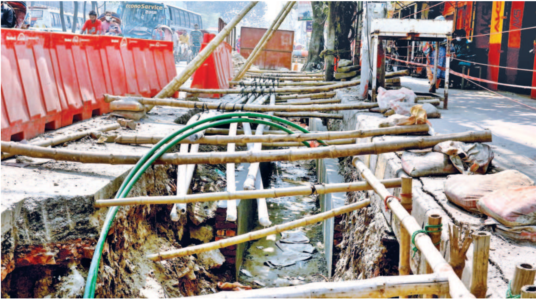
RK Mission Road at the capital's Gopibagh has been like this for months. After digging deep to facilitate drain development works, the authorities simply put up bamboos to cover the hole, while some other bamboos act as a buttress for electric poles so that they don't fall over. It goes without saying that this is immensely risky and inconvenient for the busy road's commuters. This photo was taken yesterday.
