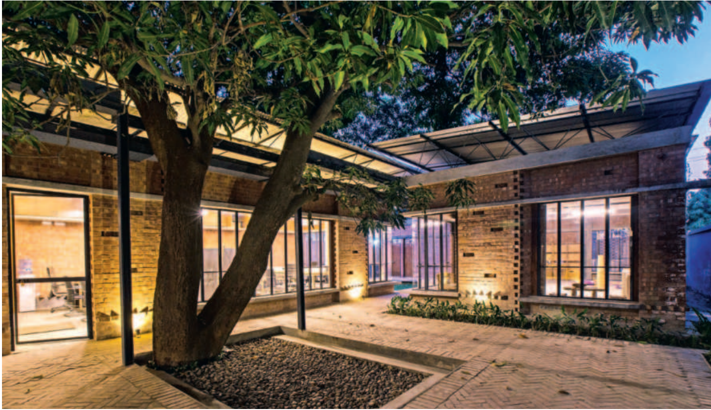
At the Teach for Bangladesh office, one will find three main pods and three service pods amid the natural setting of the premises, which consists of a mango tree, wide grass covers and neem trees. PHOTO: COLLECTED
