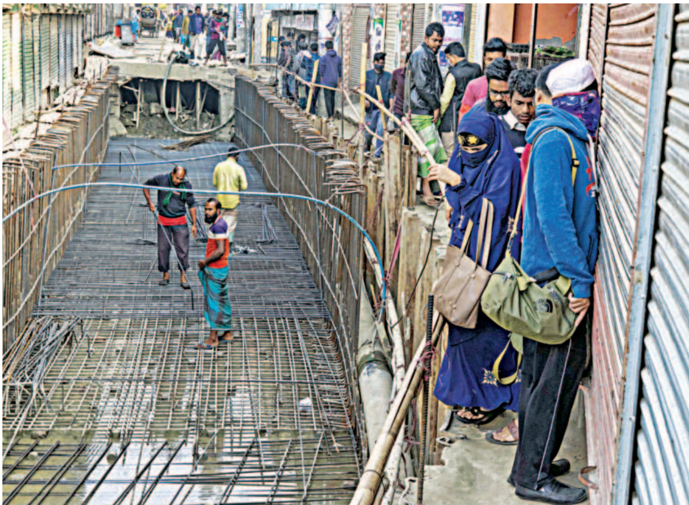
People facing difficulties crossing Chattogram city's Shantibagh area as a box culvert is being constructed without any alternative for people to cross the area smoothly. The culvert is being built for around two years under a project to address waterlogging in the port city. The photo was taken on Wednesday.
