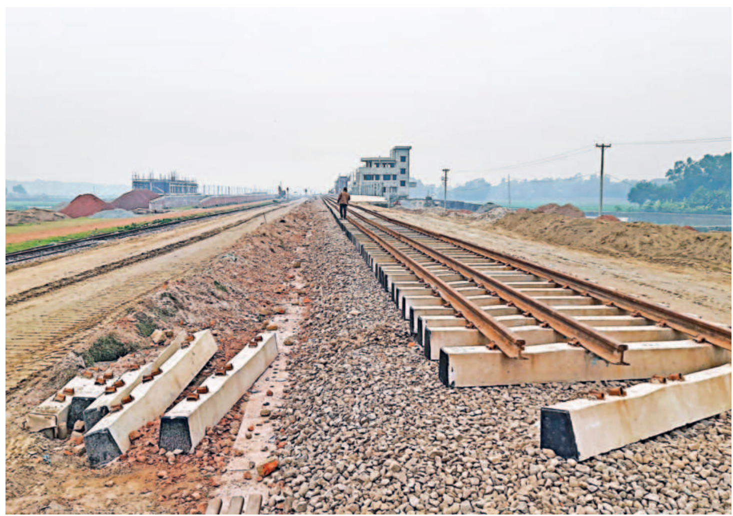
The project will convert the 225km metre gauge line into a 239km dual gauge track from Akhaura to Sylhet, helping to reduce travel time.
