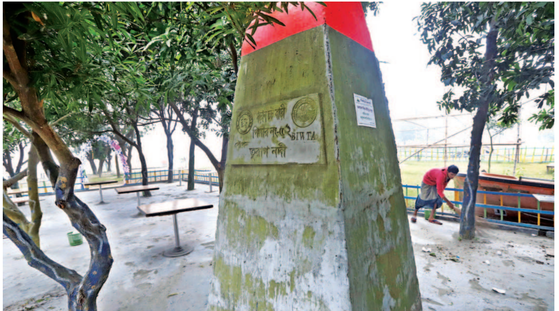
A demarcation pillar of the Turag right in the middle of a park near Botanical Garden in the capital's Mirpur area. The park was developed by a resort and entertainment centre, occupying the river's land, and the BIWTA later set up the pillar. The photo was taken a couple of days ago.
