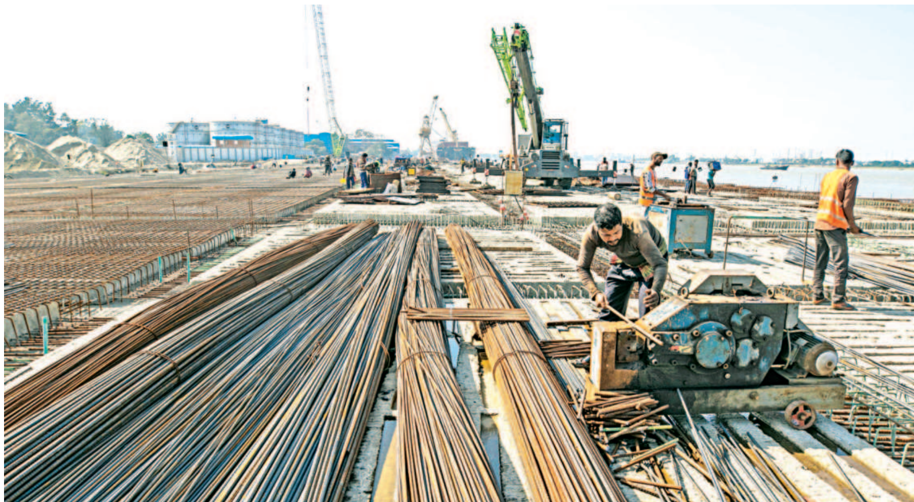
Construction of Patenga container terminal is going on in full swing through the 34 Engineer Construction Brigade of Bangladesh Army. Comprising three container jetties totalling 600 metres in length and a dolphin jetty, the terminal will be able to handle 0.5 million twenty-foot equivalent unit (TEU) containers annually. Chittagong Port Authority hopes that the new terminal would go into operation by June this year. The photo was taken yesterday.
