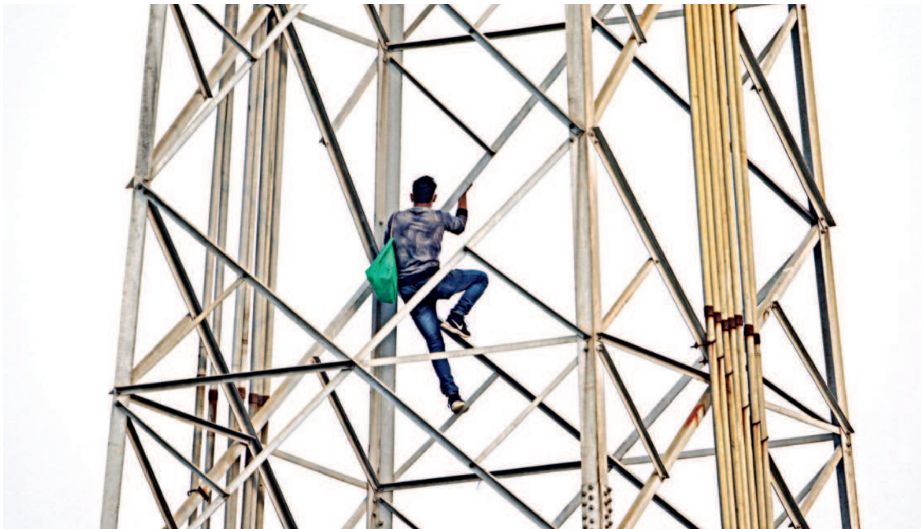
At the port city's Zohur Ahmed Chowdhury Stadium, work was underway to fix its flood lights recently. However, the workers could be seen climbing these tall structures without head gear, harness or any other kind of protective equipment, putting them under heavy risk of accidents.
