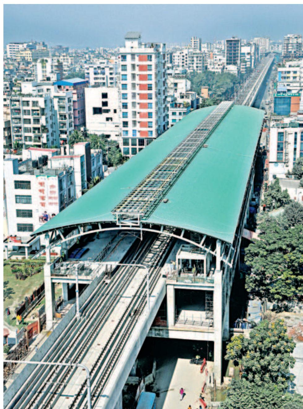
The roof trusses, which are prefabricated structures designed to support roofs, of this station of the Dhaka metro rail project were made locally by McDonald Steel Building Products. The photo was taken near Mirpur 10 in the capital recently.
