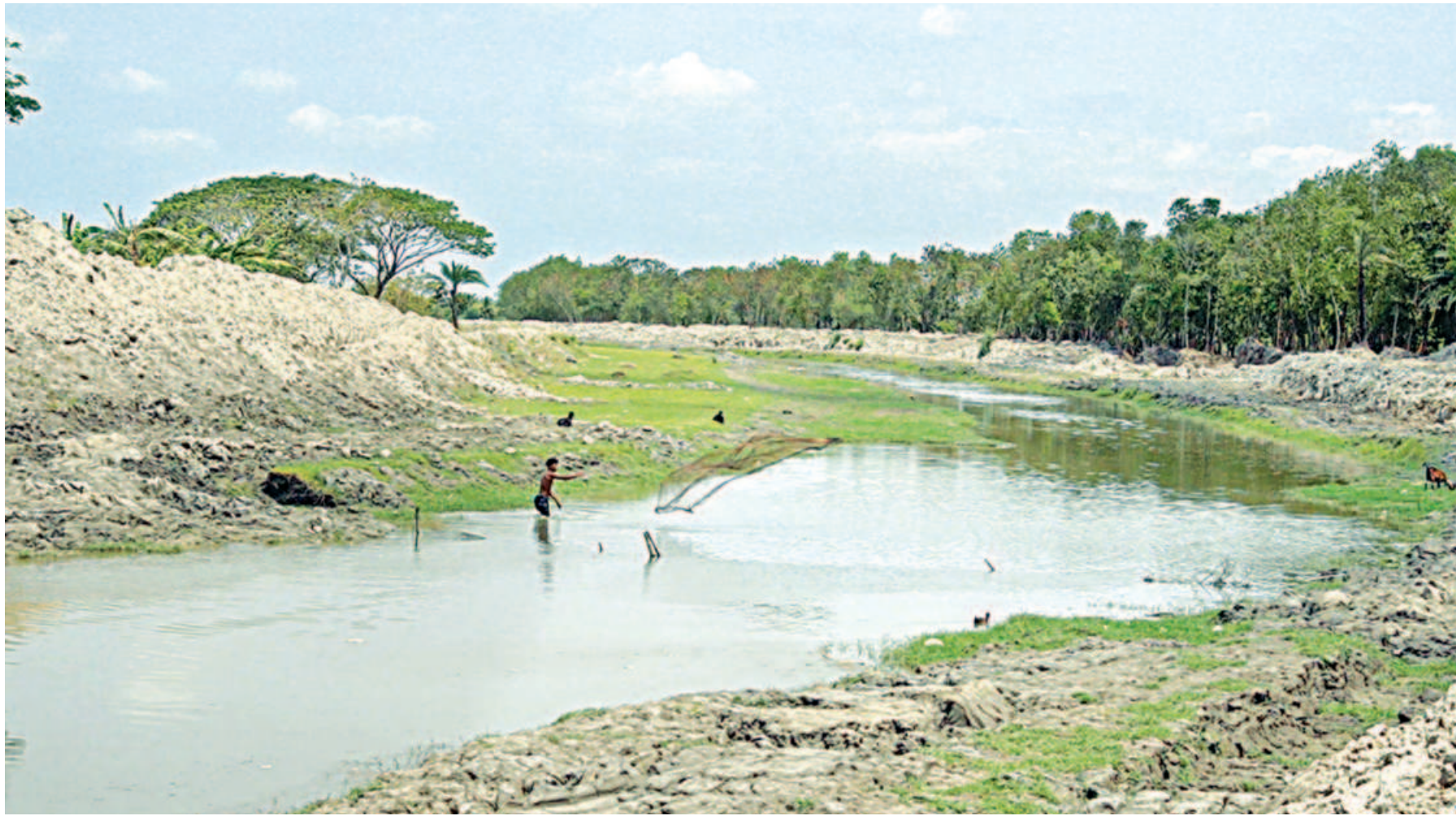
The never-ending Bhabadah waterlogging saga continues, with stories of negligence, mismanagement and even alleged corruption piling up. Beyond just people of the area, rivers such as Teka and Hari are victims to the whole situation as well. As excavated earth is dumped back onto them, both of the rivers suffer from siltation, which is raising the riverbed as well as choking the rivers' width.
