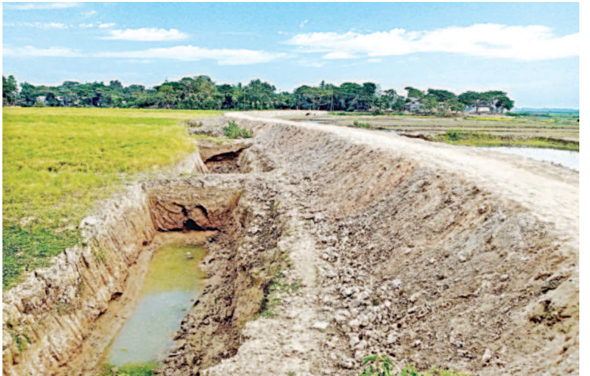
A view of the levee at Alampur village in Sunamganj's Madhyhanagar upazila. Restoration work on the levee is going on, but the dirt was taken from beneath the slope, which weakens the levee and exposes the Boro paddy being cultivated there to floods. The photo was taken recently.
