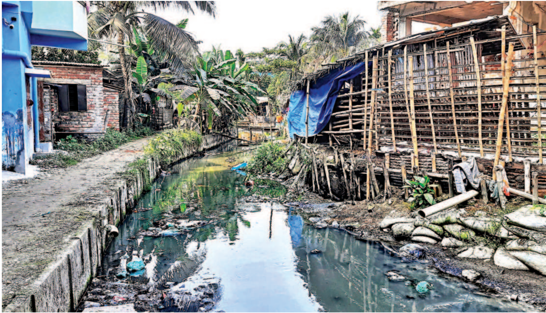
The land of this road by the banks of Taltola canal was previously a part of the water-body. But after a botched excavation, it was slowly turned into this road, which further narrowed the canal that was already plagued by waste dumping and illegal occupation.
