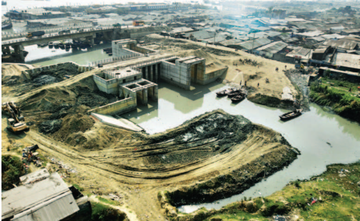
A sluice gate being installed at the mouth of the Rajarkhali canal on the bank of the Karnaphuli in Chattogram. To lessen the impacts of waterlogging, various local organisations are installing around 40 such sluice gates at points where canals in the port city fall into the river. The photo was taken yesterday morning.
