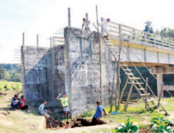
Villagers use a bamboo ladder to get into this bridge in Bandarban’s Lama upazila as there is no approach road on either side of the structure.
