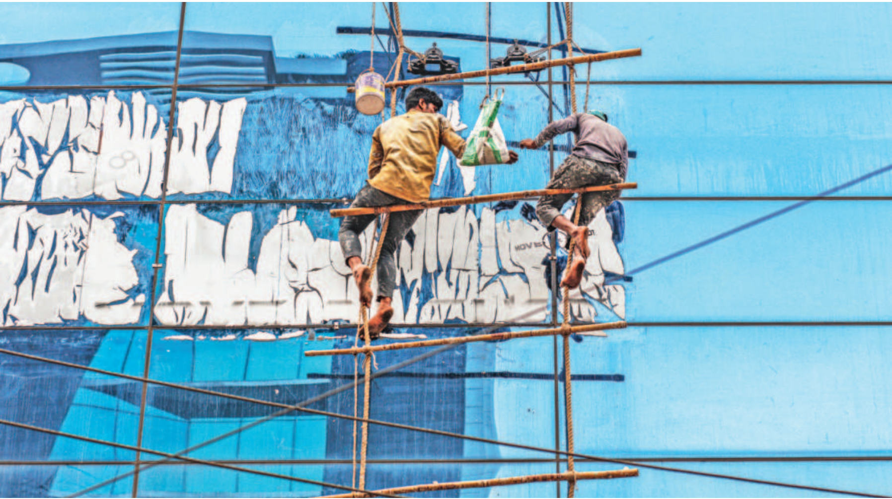
Cleaning glasses of the capital's high-rises has always been a hazardous job, which includes climbing up and hanging on to a ladder made of bamboo and rope. While the skilled workers have become quite adept at it, the process, devoid of safety measures of any kind, remains extremely risky. The photo was taken from the capital's Dhanmondi yesterday.
