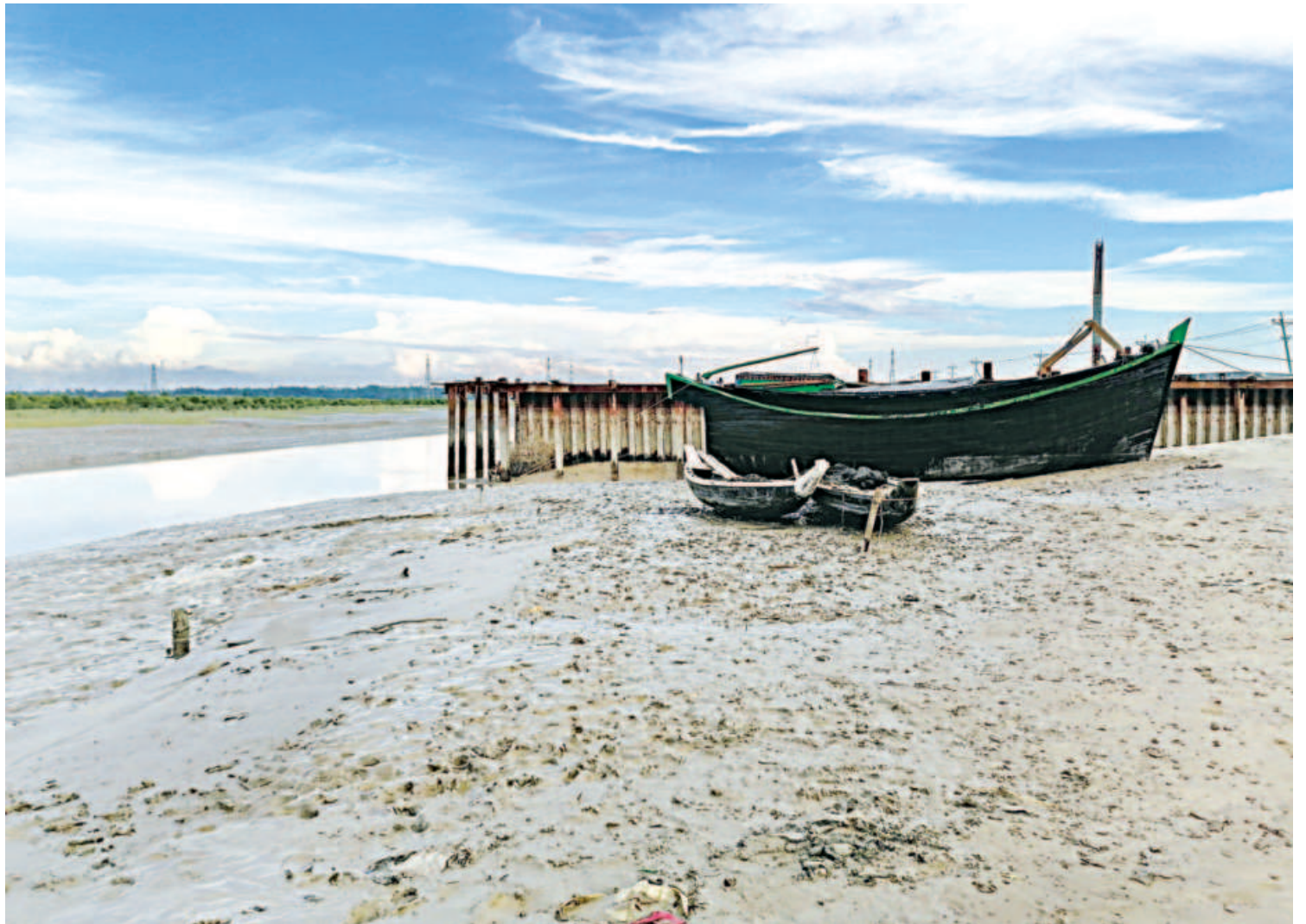
The Kuhelia river in South Rajghat area of Cox's Bazar has been narrowed due to earth-filling. The Roads and Highways Department is building a two-lane road on the river despite the land ministry's objections. The photo was taken recently.
