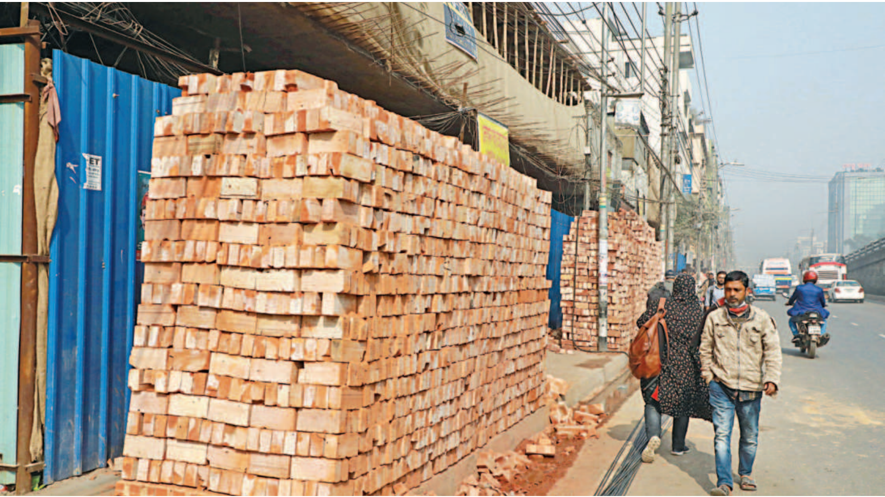
The way these bricks are piled up by this road near Mohakhali flyover are in violation of multiple laws. For one, they occupy the entire footpath, then there's the issue of leaving the bricks uncovered -- which disregards the mandate of city authorities for construction materials -- while there's also the very real risk that the stacks might collapse right on top of pedestrians at any time. This photo was taken yesterday.
