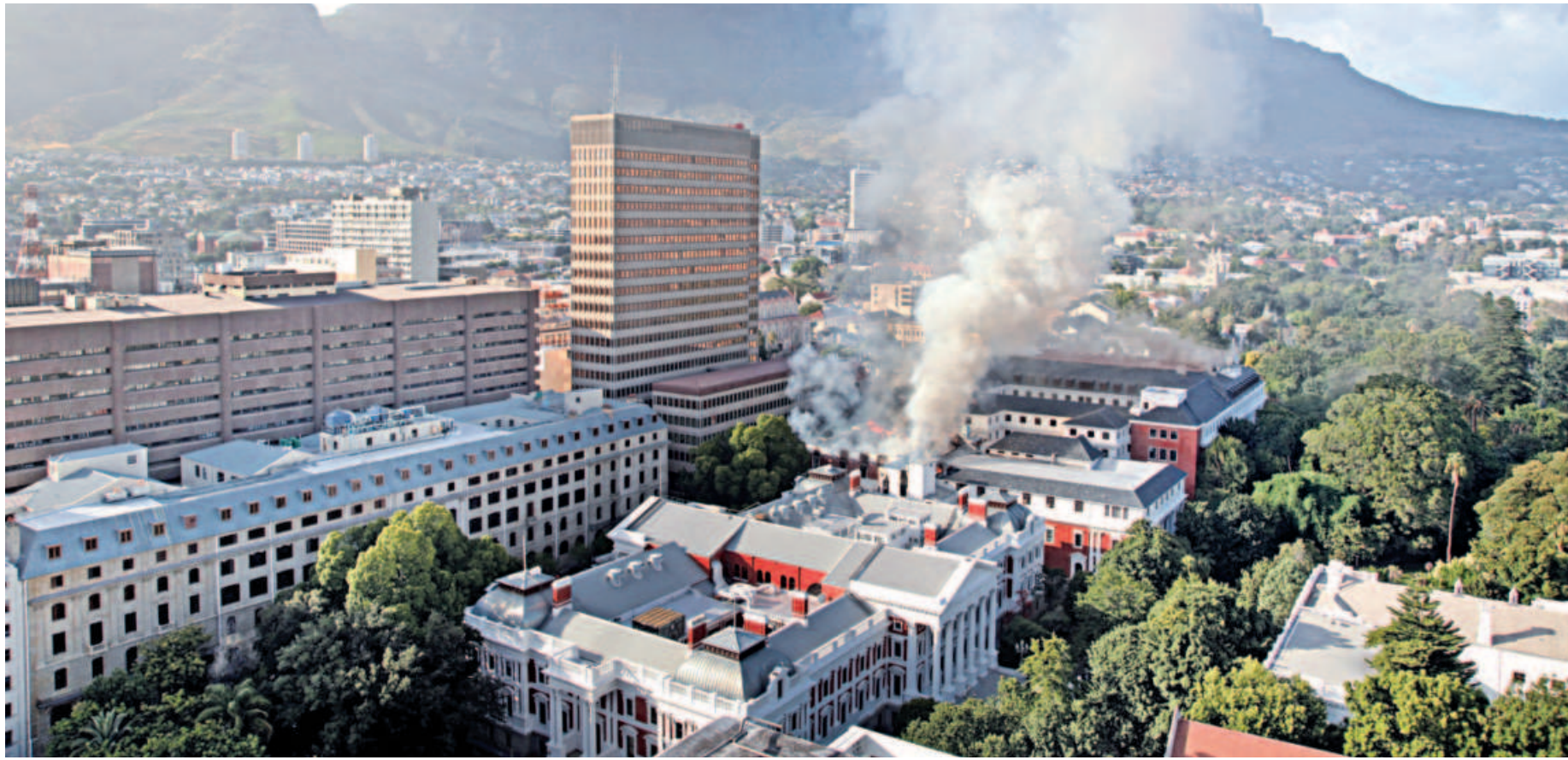
A general view of a building on fire at the South African Parliament precinct in Cape Town, yesterday. The fire caused the roof of the old National Assembly building to collapse as the blaze continued to rage after eight hours. No casualties had been reported and the cause of the blaze was not yet known.
