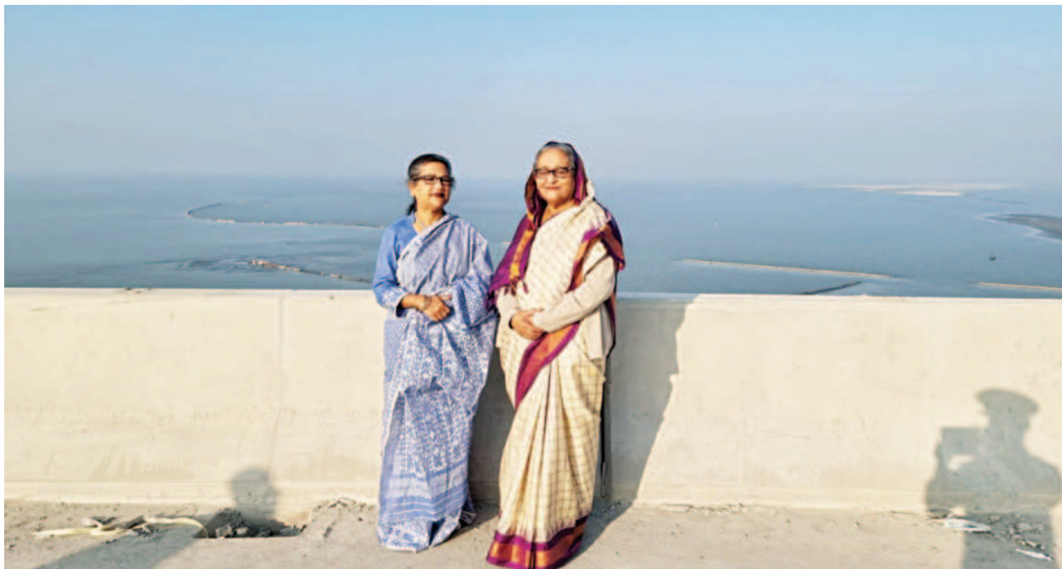
Prime Minister Sheikh Hasina and her sister Sheikh Rehana pose for a photo on the under-construction Padma Bridge yesterday morning. They took a stroll on the bridge while visiting the project site to see the progress of the work, which is nearing completion.
