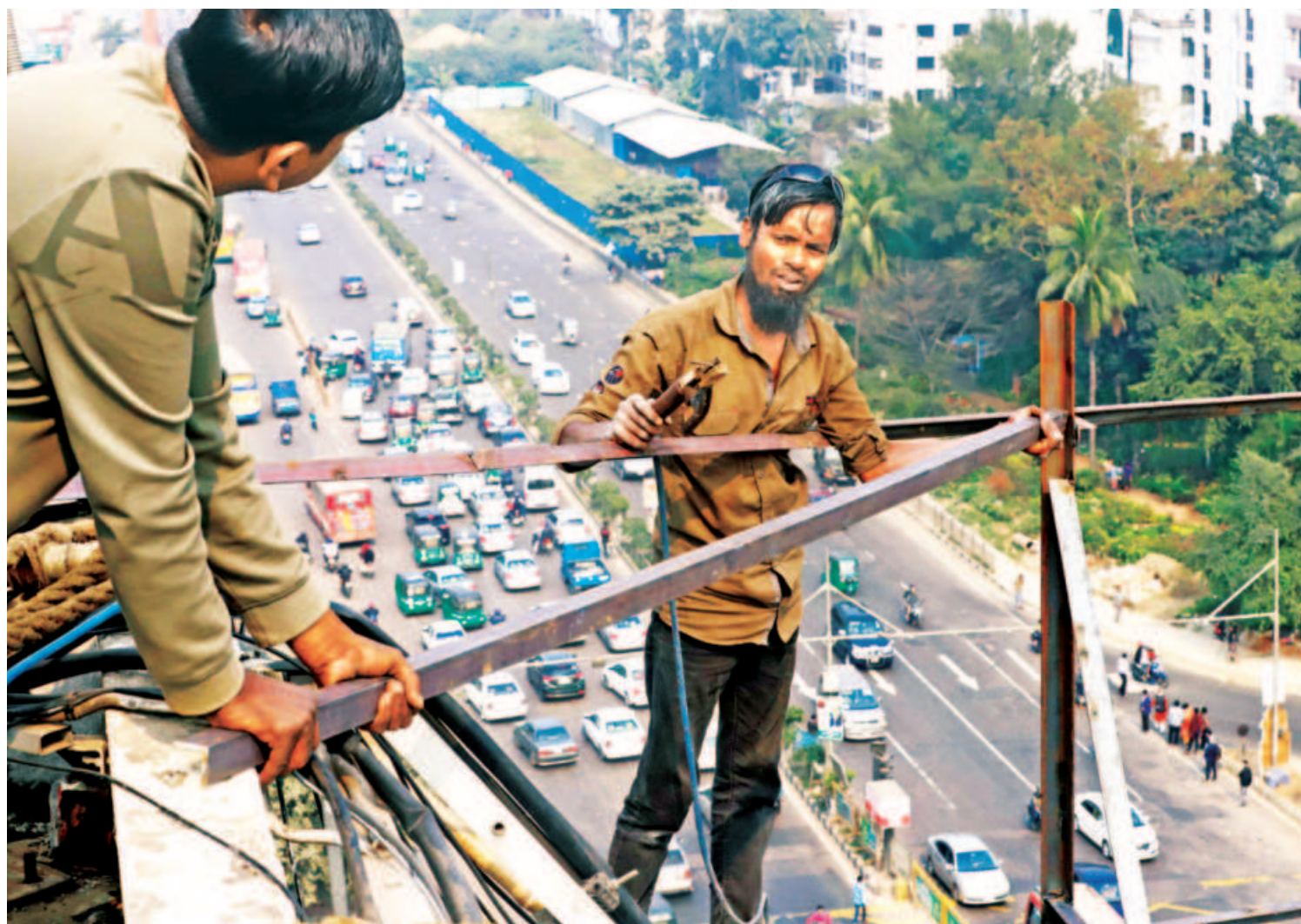
Two men are repairing a billboard at Chairmanbari in the capital's Banani area yesterday. They neither have any safety gears nor any safety harness. A little slip and a tumble from that height could be fatal.
