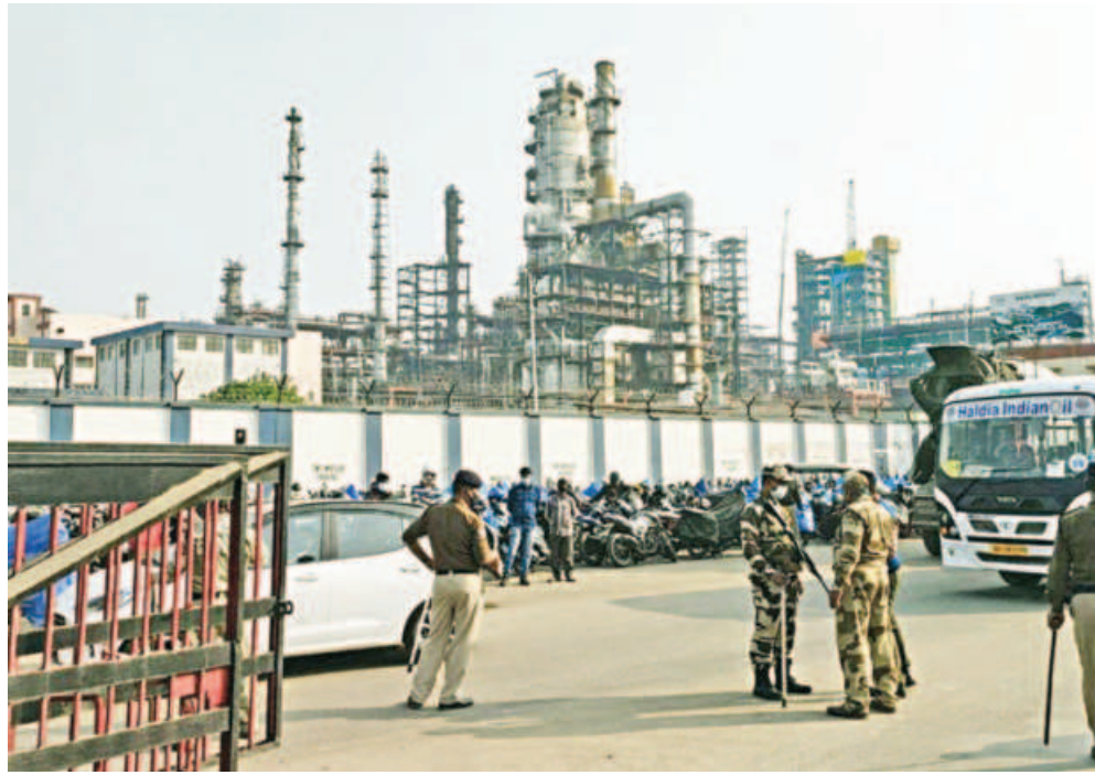
Security personnel stand outside the complex of Indian Oil Corporation's refinery in Haldia, West Bengal on December 22 a day after three people reportedly lost their lives in a fire incident in the plant.
