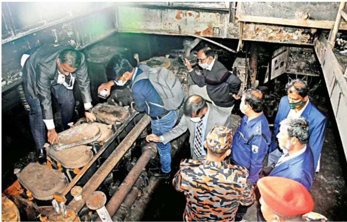
An investigation team inspects one of the engines of Abhijan-10. The engines have been claimed to be faulty, larger than permitted and installed without prior approval of the authorities concerned.
