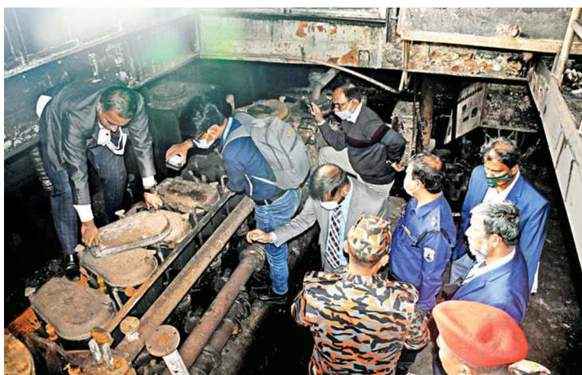
An investigation team inspects one of the engines of Abhijan-10. The engines have been claimed to be faulty, larger than permitted and installed without prior approval of the authorities concerned.
