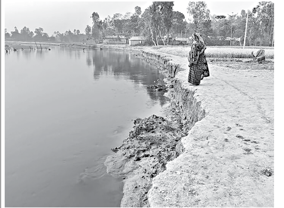
Arable land and homesteads are being devoured by unabated erosion of Teesta even in the winter. The photo was taken from Gatiyashyam village in Gharialdanga union of Kurigram's Rajarhat upazila recently.
