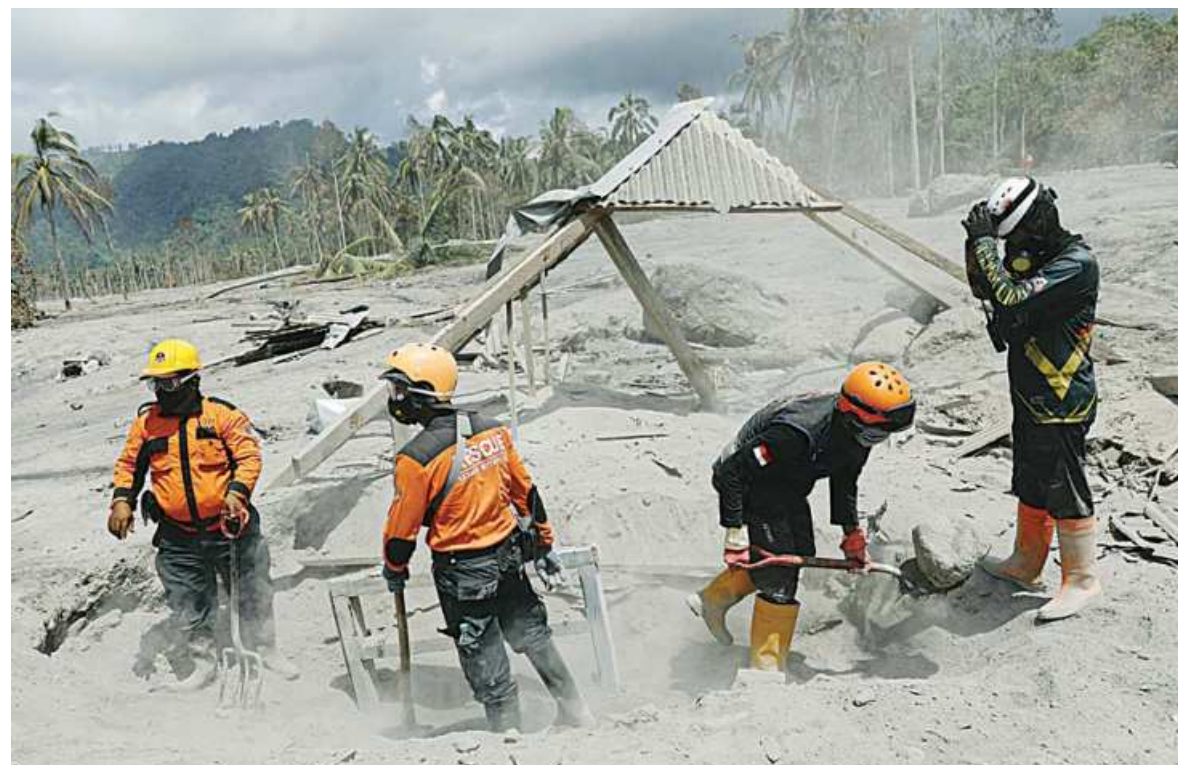
Rescuers dig a damaged building during an operation at an area yesterday which was affected by the Mount Semeru volcano eruption that killed at least 43 people last Saturday in Sumberwuluh, Candipuro district, Lumajang, East Java province, Indonesia.
