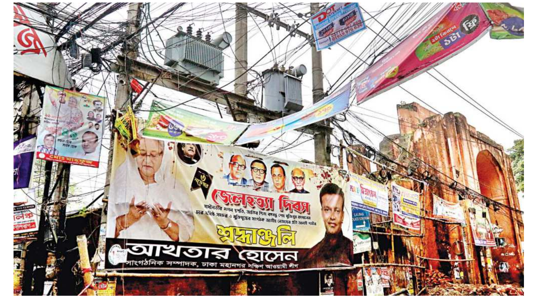
Banners hanging from electricity poles and tangled webs of cables mar the beauty of the entrance to Lalbagh Fort, an architectural jewel of the Mughal Empire, in Old Dhaka. The photo was taken yesterday.
